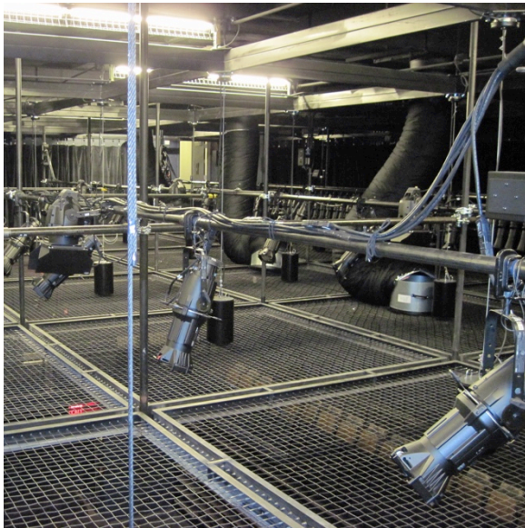
Figure 8 Tension Wire Grid
